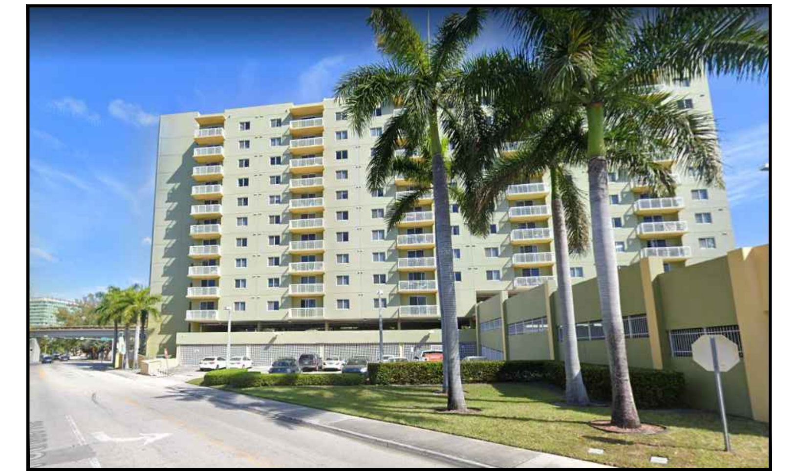
BUILDING AT SE OF SITE
