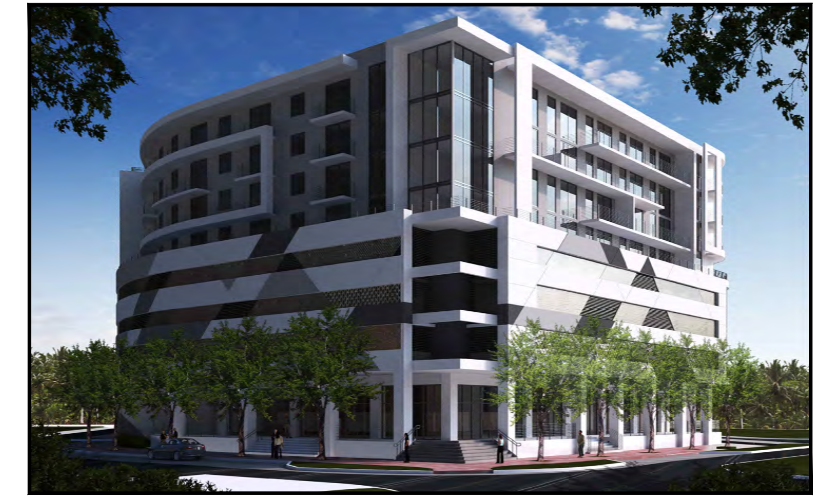
BUILDING AT NORTH OF SITE (SOLESTE SPRING GARDEN / UNDER CONST.)
